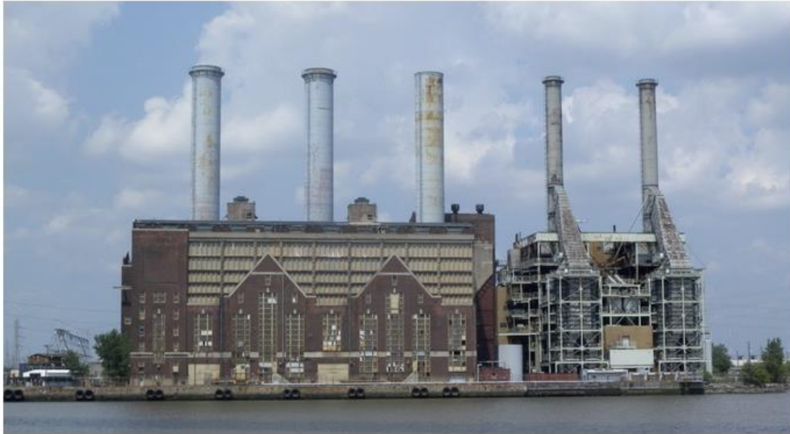
The Kearny Generating Station in a gas peaker power plant in New Jersey. It comes on when AC use spikes the electricity grid.
